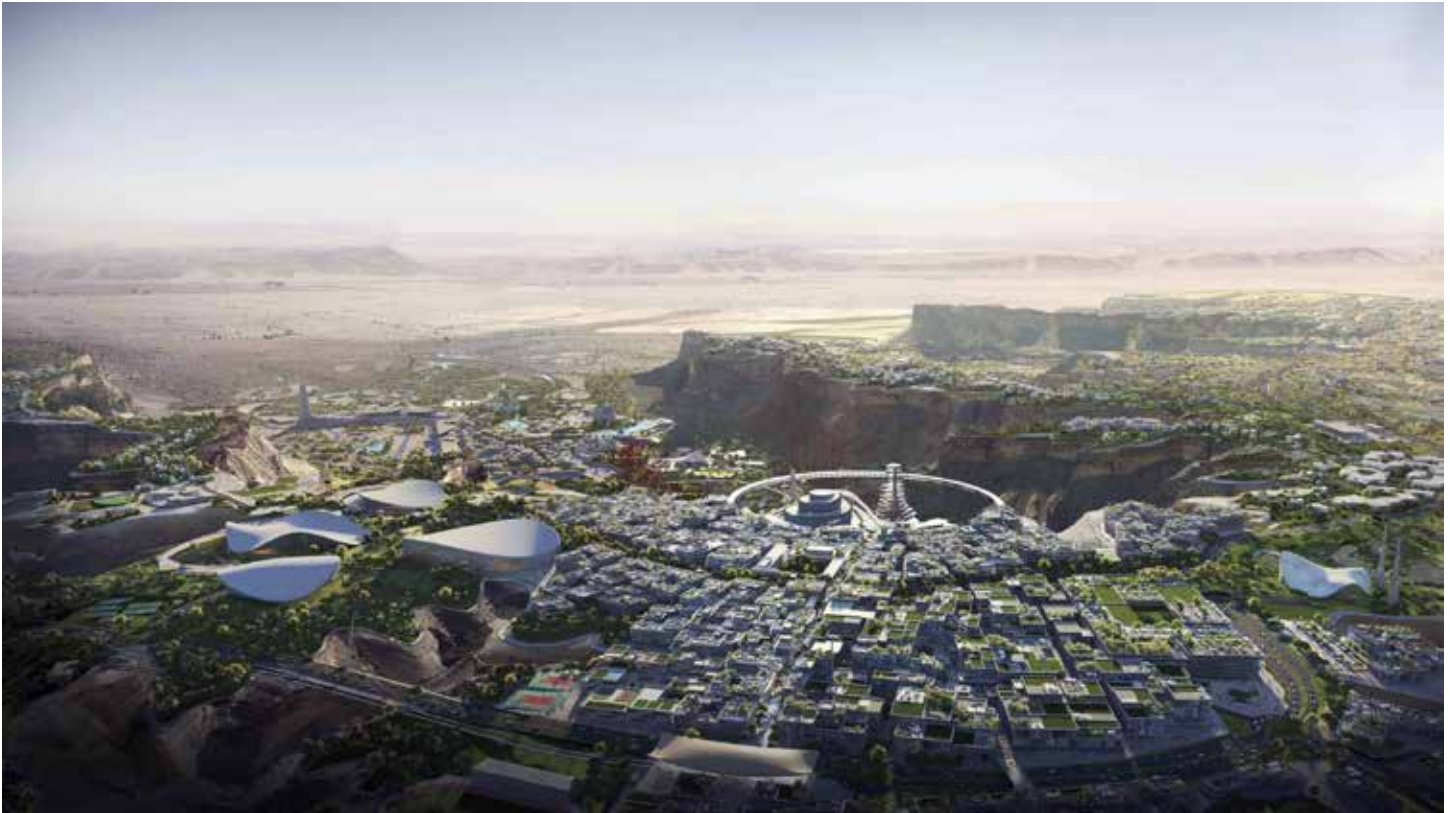
The construction of Qiddiya, an entire city dedicated to play, is an example of the investment in entertainment licensing in the Middle East.
